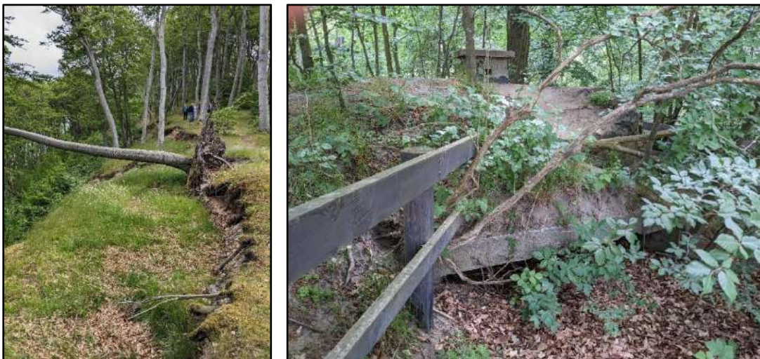
Cliff top slump and sandy accretion around bunker
